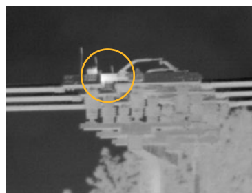
Figure 6. This third image of the substation transmission line, captured with a Fluke 4x telephoto lens clearly shows a hot spot or high resistance on a knife switch.
